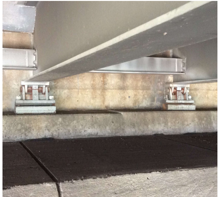
PHOTO 2 Description Bent 1. Bearings at beams 3 & 3. Fretting.
