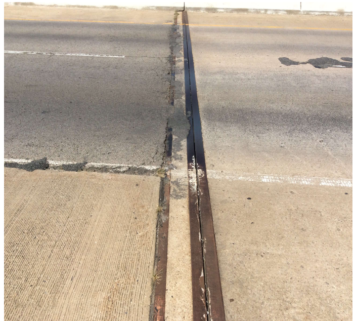
PHOTO 2 Description Bent 1. Expansion joint
