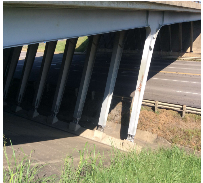
PHOTO 5 Description Bent 2, Beam 6. Corrosion.
