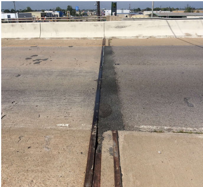
PHOTO 1 Description Bent 4. Expansion joint
