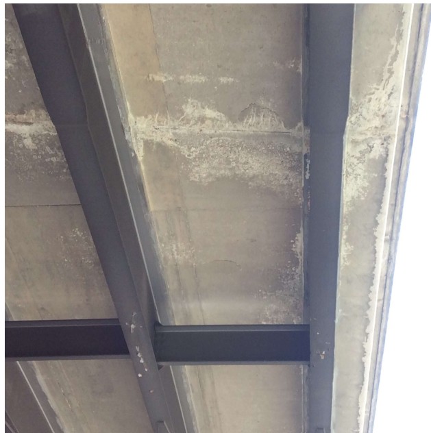
PHOTO 4 Description Delaminated areas over Eastbound lanes.
