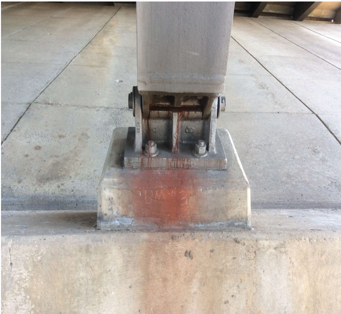
PHOTO 1 Description Bent 3. Column 3. Fretting
