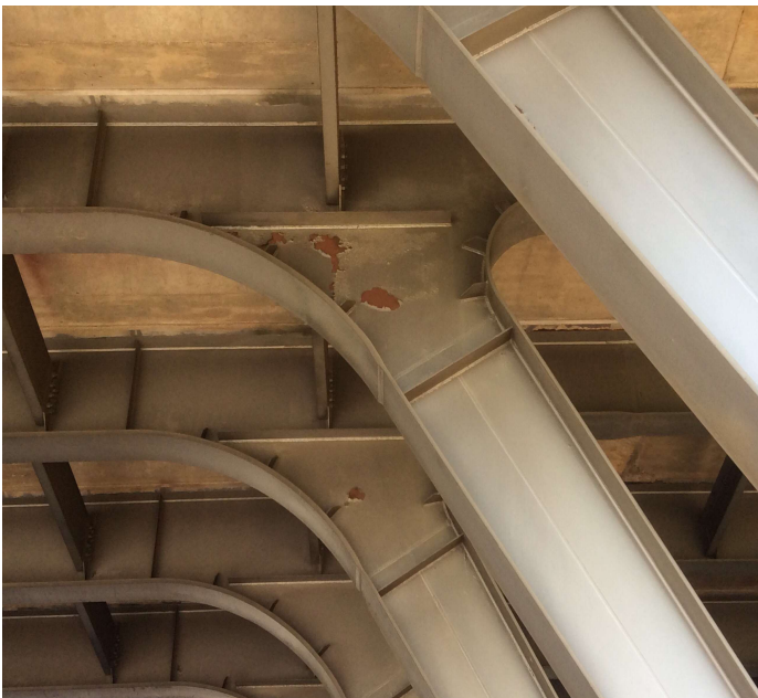
PHOTO 1 Description Bent 3. Column 3 & 4. Paint peeling.
